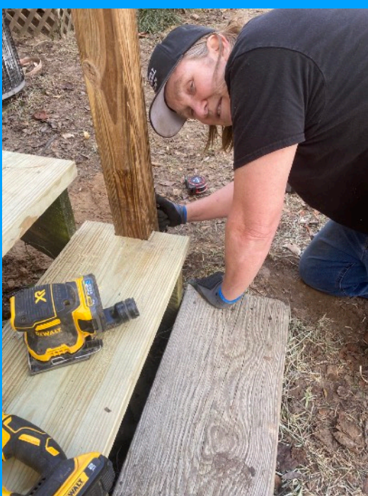
Marko repairing a friend's stairs
